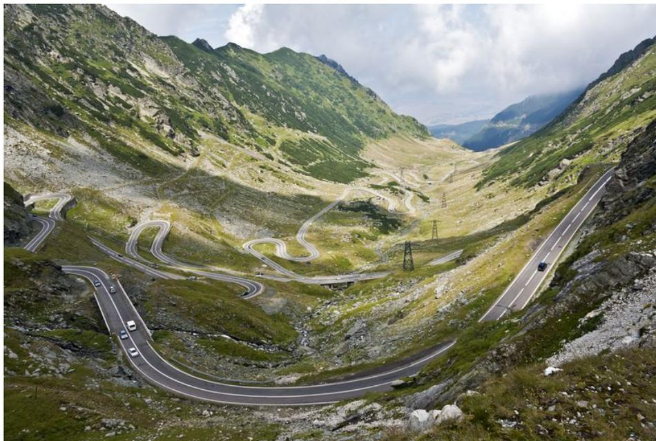
The highway above switches back and forth as it climbs up the steep hillside. The much gentler slope of the road makes it easier for vehicles to reach the top of the mountain. The highway is an example of an inclined plane.
